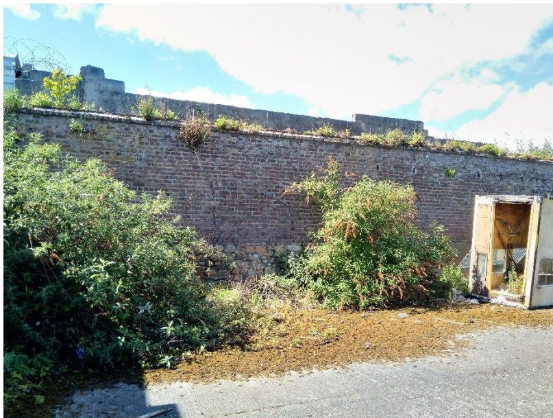
FIGURE 5. BRICK WALL AT THE SITE OF THE PROPOSED DEVELOPMENT. (IMAGE TAKEN 07/05/2021).
