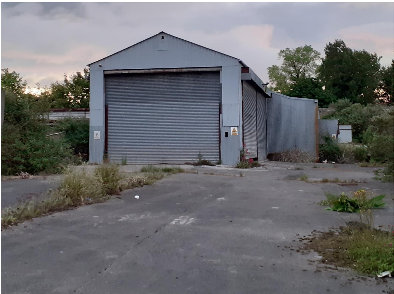
Plate 4: Example of corrugated building within the proposed development site.
