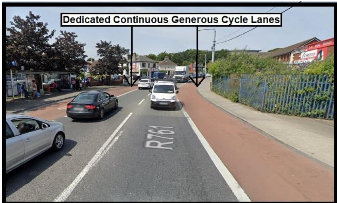
Figure 2.1 – Pedestrian & Cycle Facilities in Place at Castle Street
