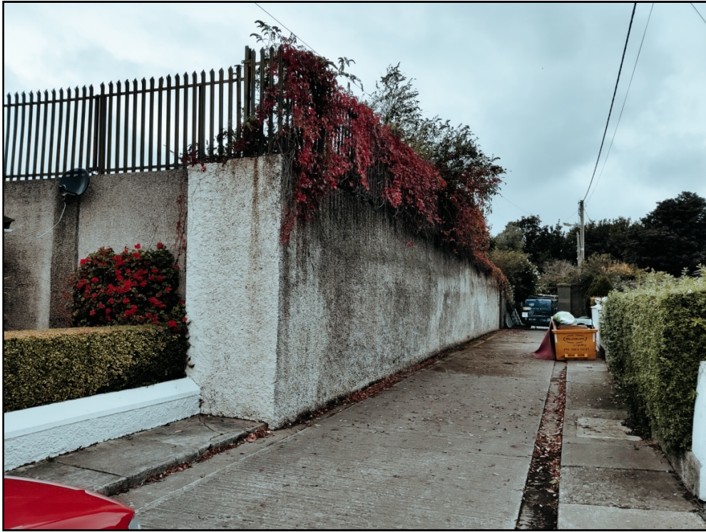
Plate 12 View of the boundary wall B, from the exterior, looking NW.
