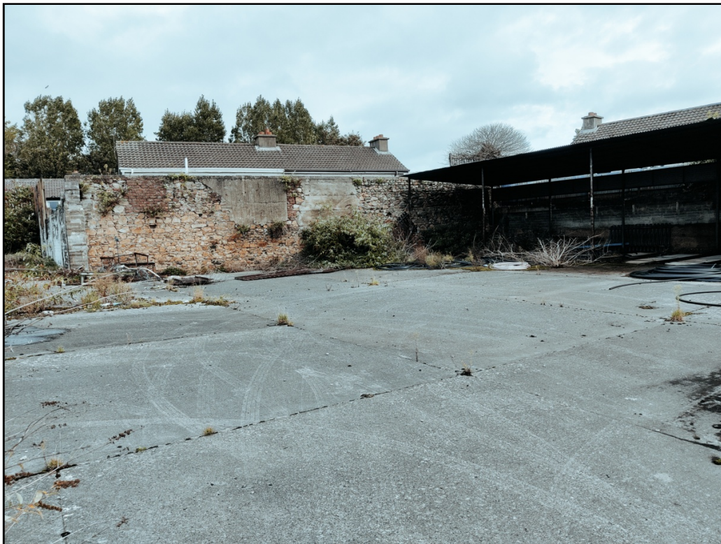
Plate 5 View of north-eastern yard, looking NE.
