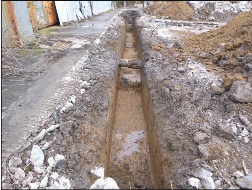
Plate 28 Trench 6, looking NE.
