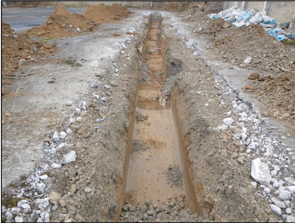
Plate 20 Trench 2, looking NE.
