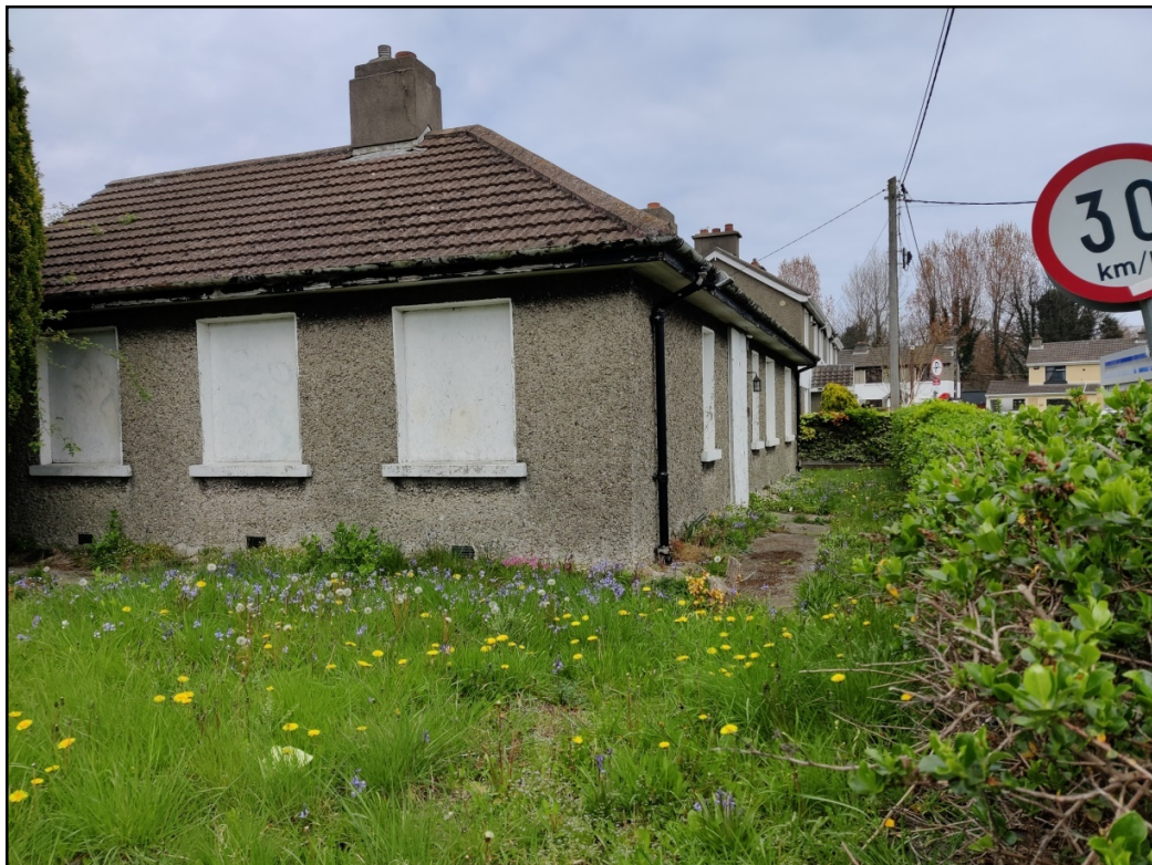
Plate 9 No. 20 Dwyer Park (III), looking NNW.
