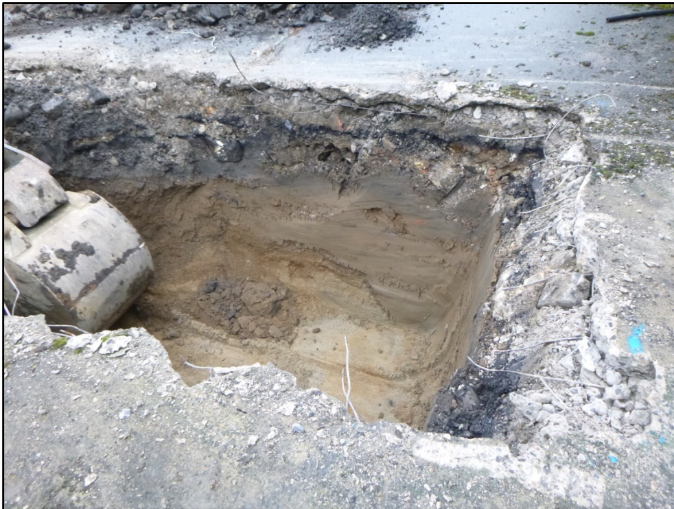
Plate 30 Trench 7, looking NE.
