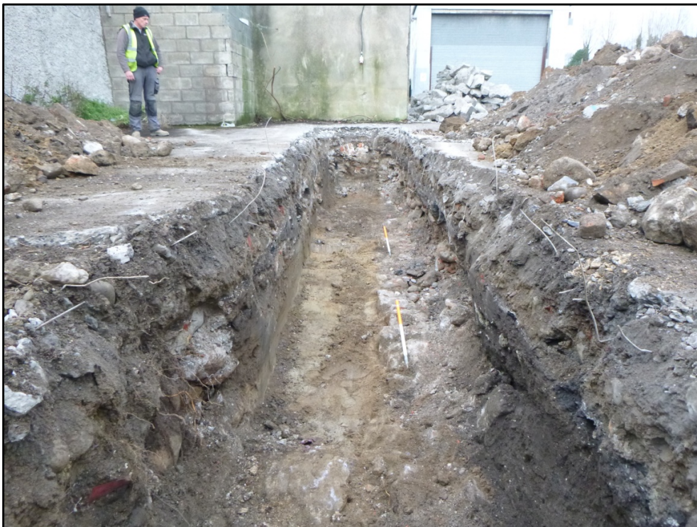
Plate 25 Trench 4, looking NE.
