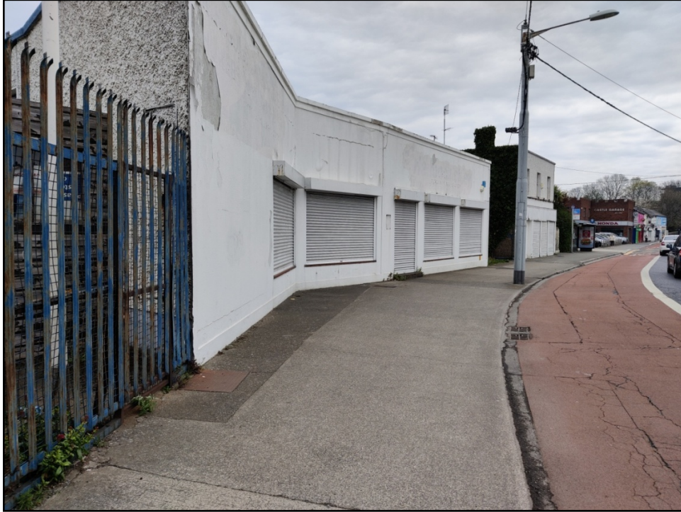
Plate 2 View of former showroom/shop building fronting Castle Street, looking E.
