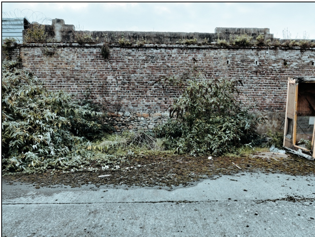
Plate 13 View of the boundary wall C, looking SW.
