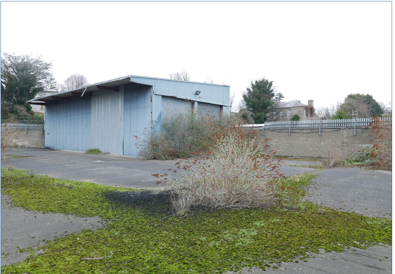
General View of the north east corner of the site.
